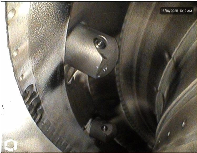
General view on leading edge of Combustion liner.
